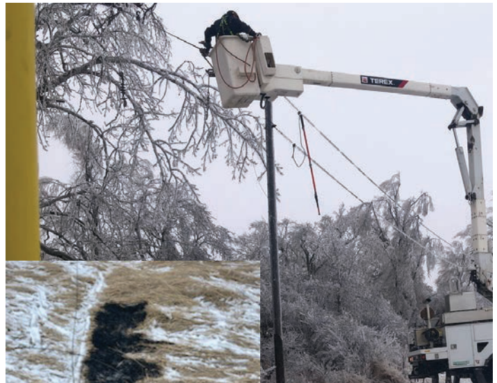
Above: Crews remove heavy ice covered trees from lines.
