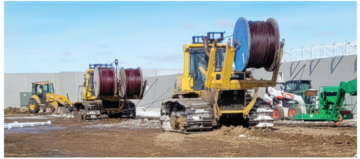
Above: Crews are burying underground for Plainview Colony's new hog barn.
