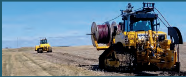
Work commenced in the Eureka area in late April as FEM's contractor began to plow in underground line.
