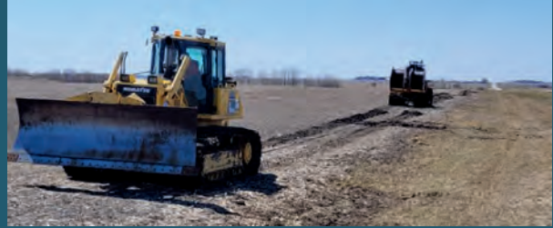
Work commenced in the Eureka area in late April as FEM's contractor began to plow in underground line.
