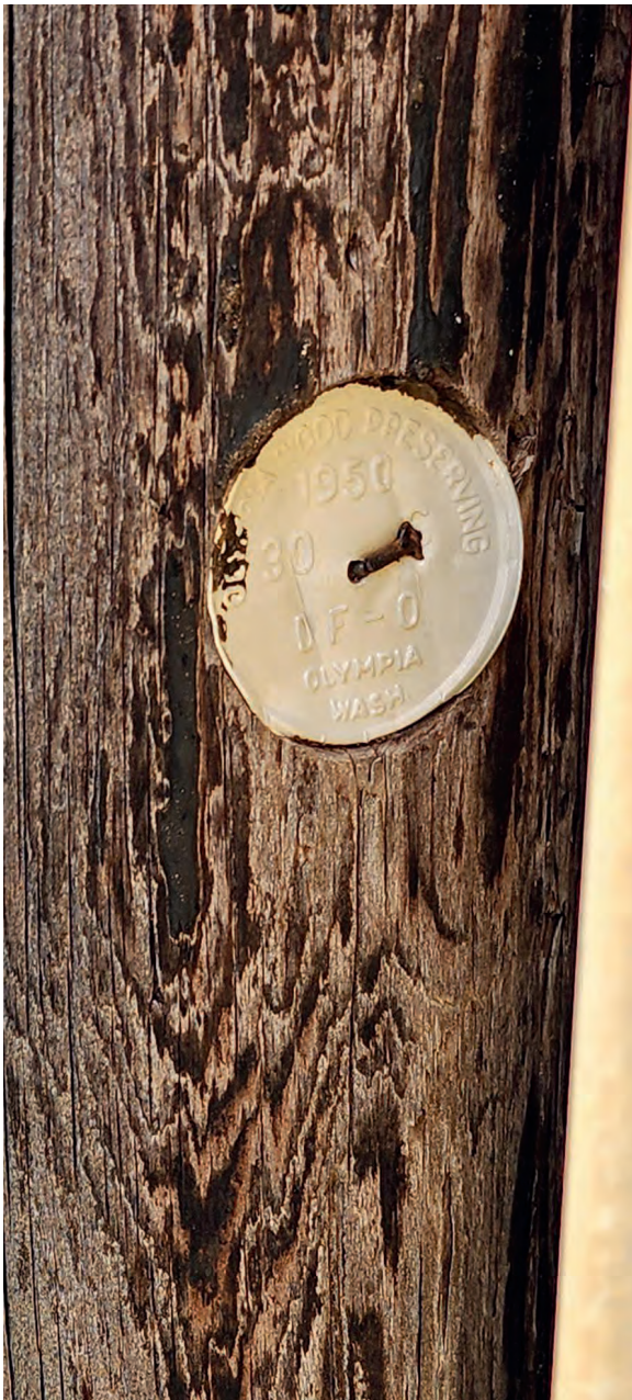
One of the original utility poles on Ken and Kathleen Meier's land was created in 1950, yet it still functions to this day.
