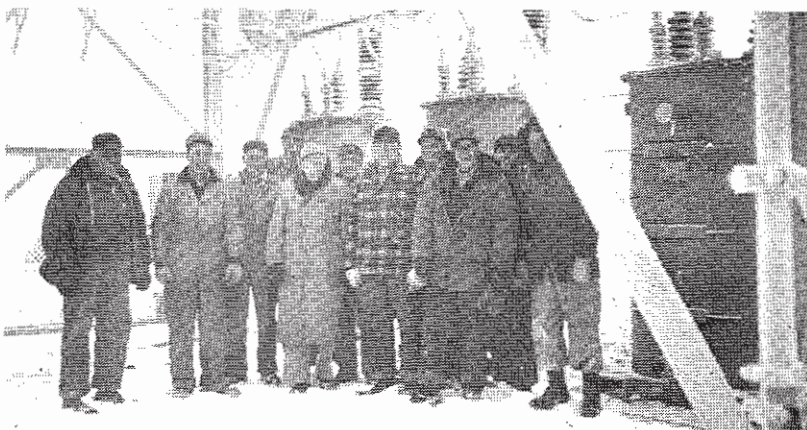
When the last of the three initial substations, the Tolstoy Substation, was energized on December 19, 1949, service was provided in all three counties, thus establishing the back bone of FEM's distribution system.
