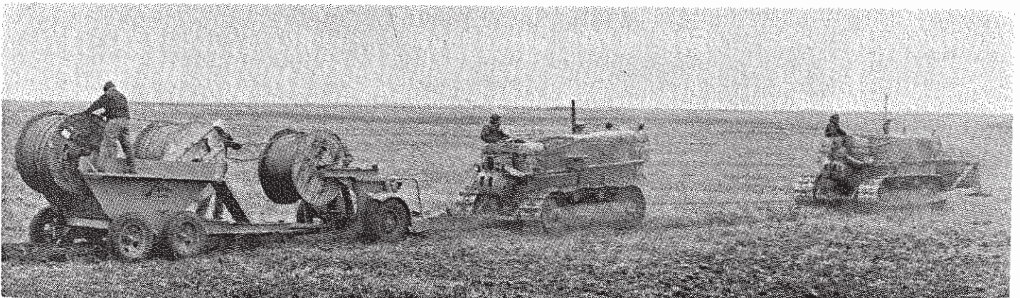
FEM's first underground was installed in 1969 preparing for the construction of the Newtown Substation.
