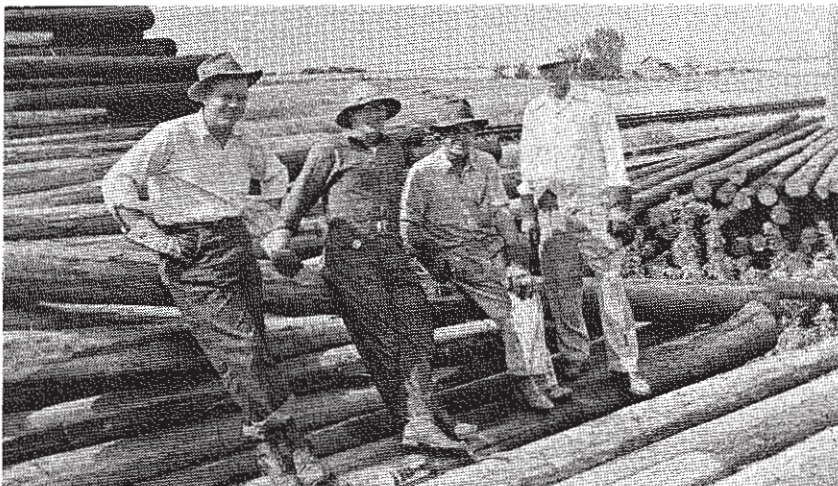
During the early years, poles were shipped by rail and stored near the tracks. FEM employees Dick Bosanko, Walter Koth, Glen Brown, and Allie Graze take a break from loading poles.
